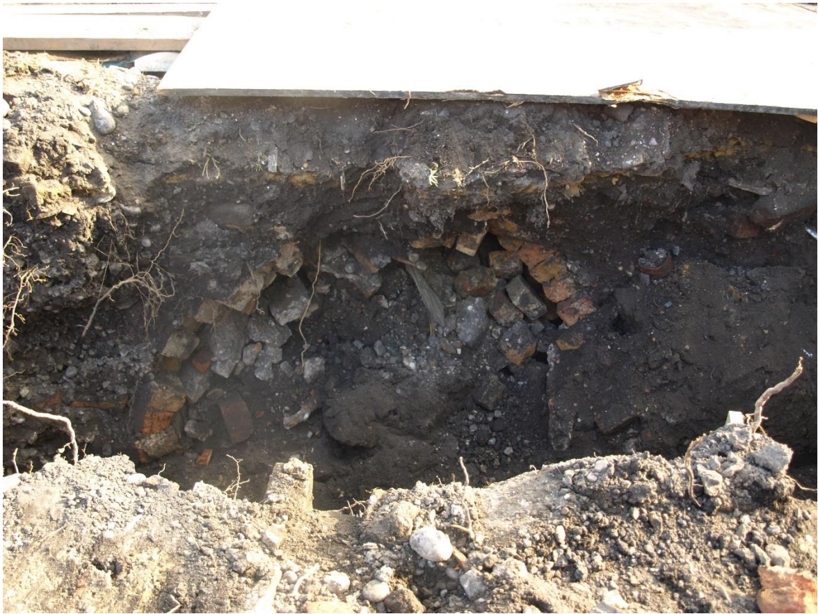
Plate 8 Culvert (004), viewed from the north
